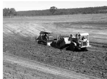
New water infrastructure, Mimosa Station, QLD.
