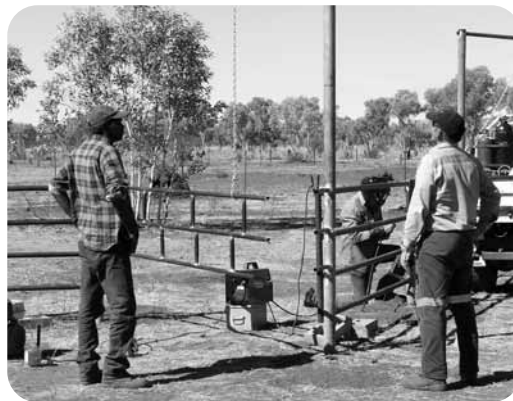
Building a spear trap cattle yard on Lamboo Station.
